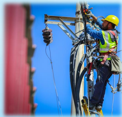
Added Low Voltage Network lengths 748.8 KM
